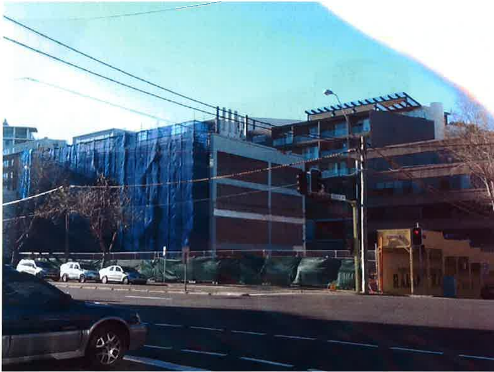
Figure 3. Current view of the site (from southern cnr. of Pacific Hwy & Oxley St)
