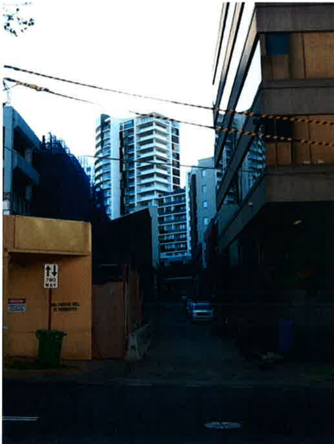
Figure 4. View of Clarke Lane (from Oxley Street)
