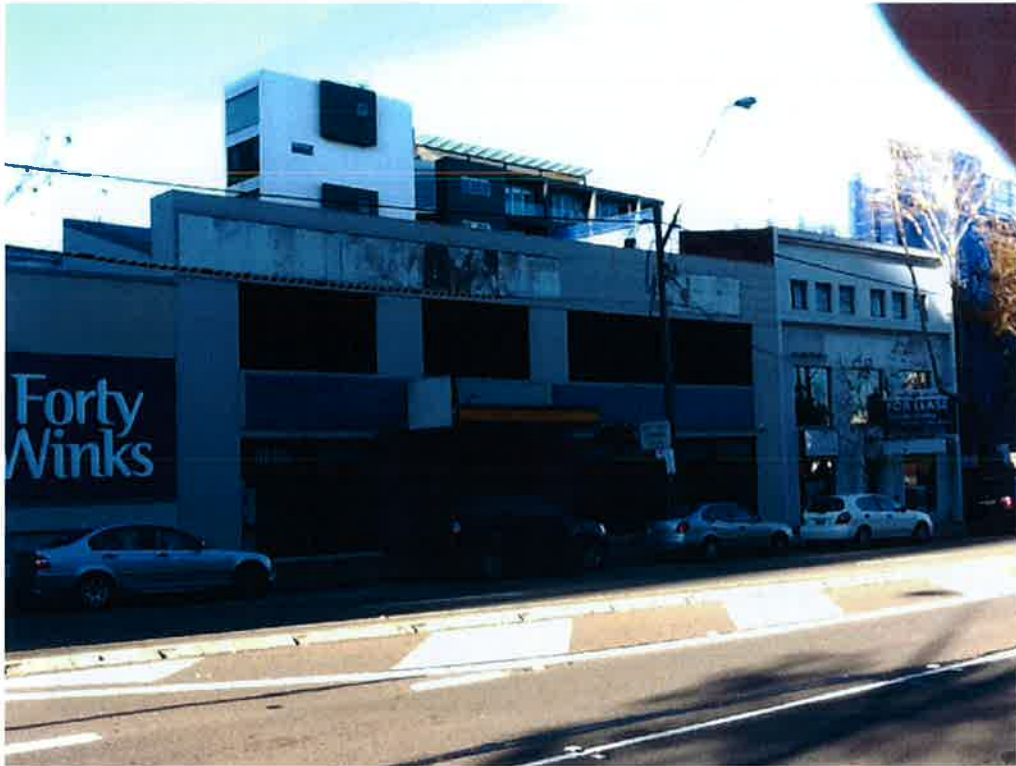
Figure 5. View of adjoin buildings immediately north west of the subject site
